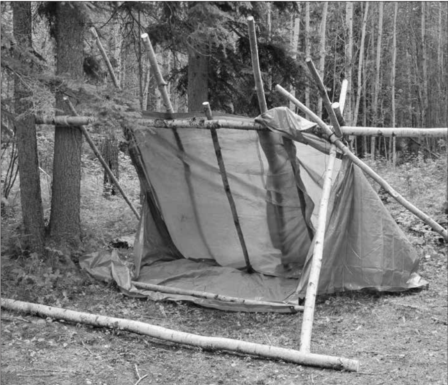
A common lean-to using tarps for the roof and ground sheet. This example, although functional, has major weaknesses with no ground insulation and the overly large opening allows heat to escape. It does provide great practice of construction techniques and is taught at most beginner camps.
